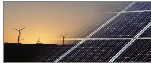
Solar PV and Wind Infrastructure
